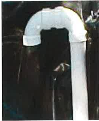
Figure 1 Basic Vacuum Vent
