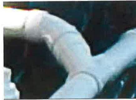
Figure 3 Vent Branch Connection
